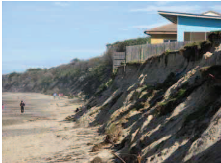
Figure 3.1. Erosion at Old Bar, Taree (7 July 2008).
