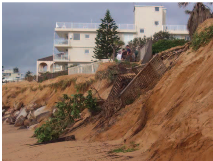
Figure 4.2. Coastal erosion at Collaroy/Narabeen beach (June 2007).
