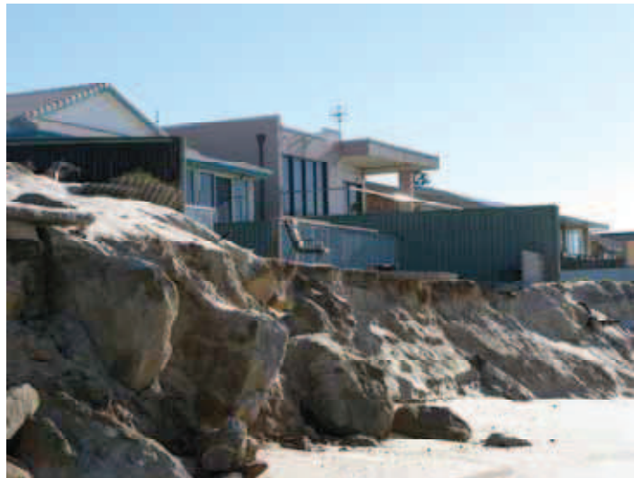
Figure 4.1. Erosion at North Entrance, Wyong Shire (12 June 2009).
